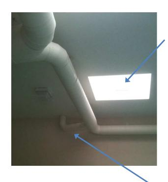
Though barely visible in this photo, a supply register was piped into each sky light box to stops the perpetually forming condensation on the skylight.
