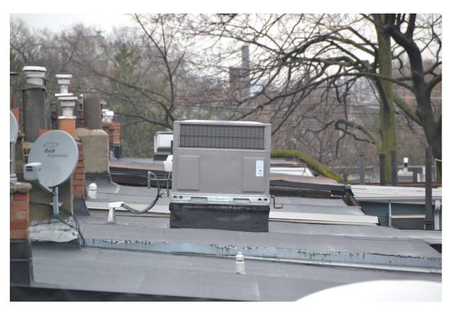
This roof top furnace and A/C system was installed because the owner didn't want unsightly bulkheads/drop soffits inside.
