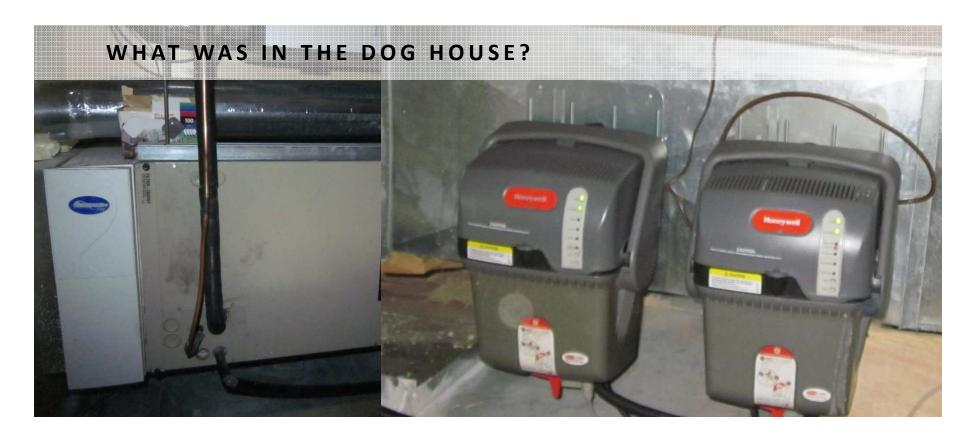
An A/C air handler and a pair of Honeywell steam humidifiers (note leak on right unit).
