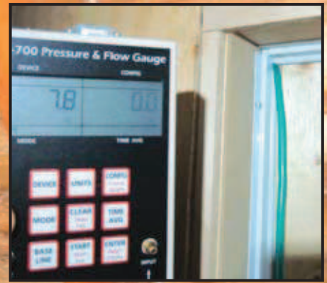
Photo 2: 7Pa of pressure in the dog house driving the moist air into the attic
